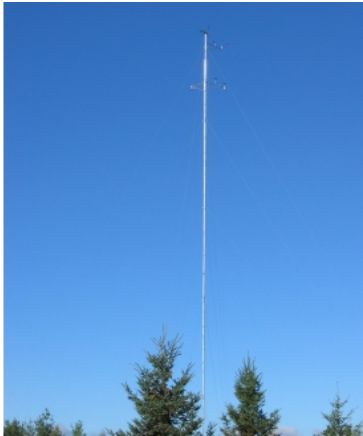
Air X on a 122 foot tower with an anemometer at hub height
